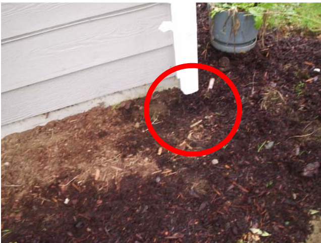
Install splash block right rear of house
